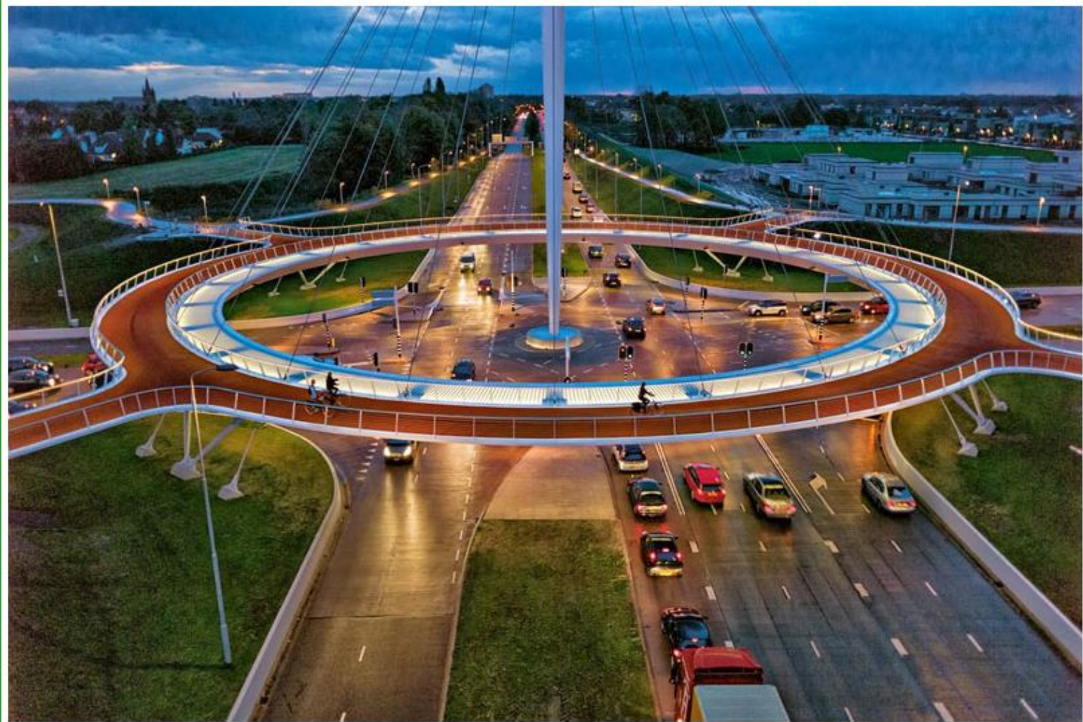
“Hovenring” suspended bicycle roundabout in Netherlands ( twistedifter.com 1-30-14)
